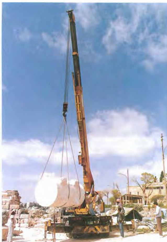
The lifting of the first drum (a newly-cut one). Photo by Anthi Koutsoukou.
