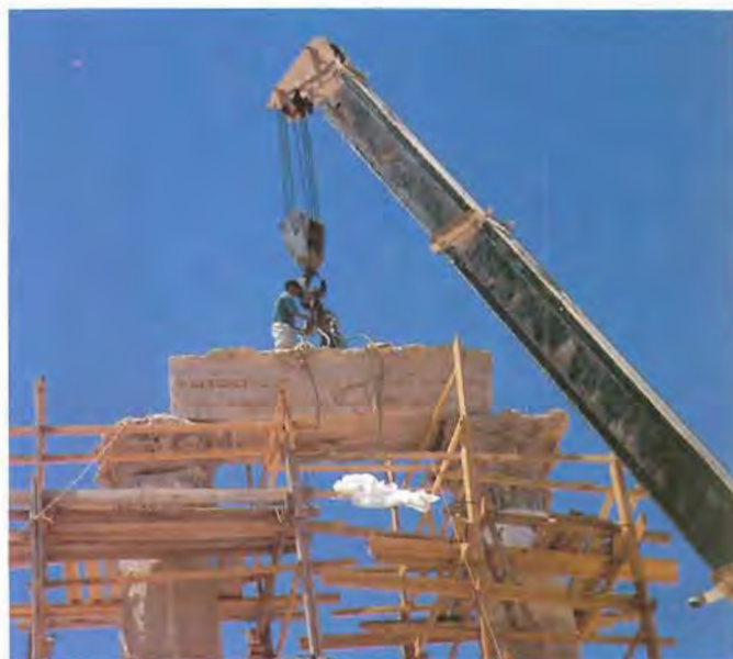
The architrave being set in place. Photo by Anthi Koutsoukou.
