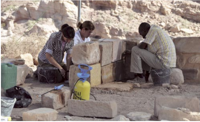
TWLCRM Lead Conservator Christina Danielli (center) and conservation technicians Mohammed Freij (right) and Milena Zafirova (left) build a new wall for testing different lime mortar mixtures; photo by Qeis Twaissi
