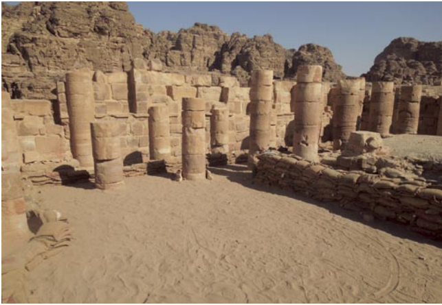
The temple interior (cella) after completing the temporary, protective backfilling of the floor and the building of sandbag barriers around sensitive features; photo by M. Elena Ronza
