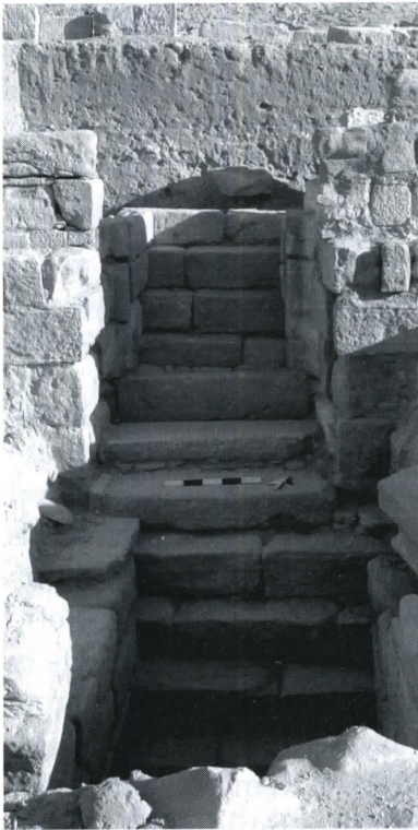
The steps between the two sections of the complex
