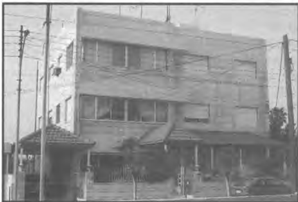
ACOR near the Fifth Circle; 1977-86
