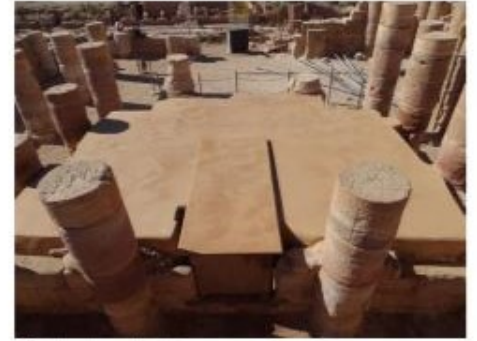
protective mortar capping on the cella podium (photos by Franco Sciorilli)
