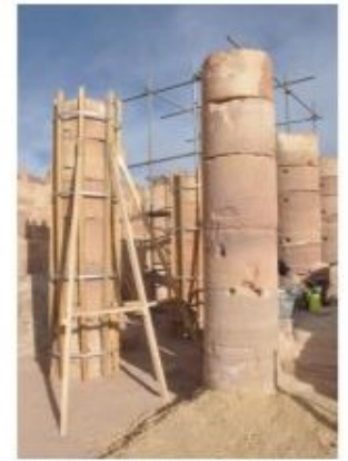
Side view of cella undergoing work led by Lead Conservator Franco Sciorilli with senior conservation assistant Hamza Wakhyan (left); conservation assistant Halemah Nawafleh applying mortar to a column (center); and one of the leaning columns after the addition of a wooden structure (right) (all photos by TWLCRM team)
