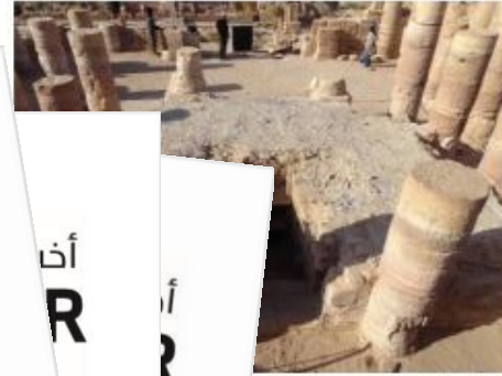
protective mortar capping on the cella podium (photos by Franco Sciorilli)
