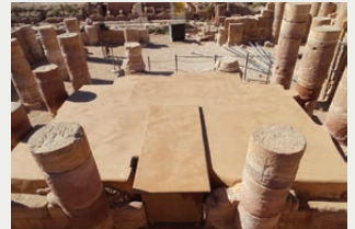
Work by conservator Franco Sciorilli included the 2017 addition of a protective mortar capping over the exposed temple podium in the cella.
