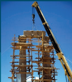
Reconstructing columns in the “Temple of Hercules” on the Amman Citadel
