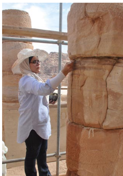
Columns in the west side of cella undergoing work led by Lead Conservator Franco Sciorilli with senior conservation assistant Hamza Wakhyan (left); TWLCRM documentation assistant Halemah Nawafleh applying mortar to a column (center); and one of the leaning columns after the addition of a wooden bracing structure (right) (all photos by TWLCRM team)
