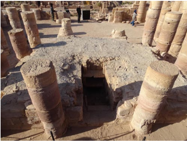
Before and after the application of a protective mortar capping on the cella podium (photos by Franco Sciorilli)
