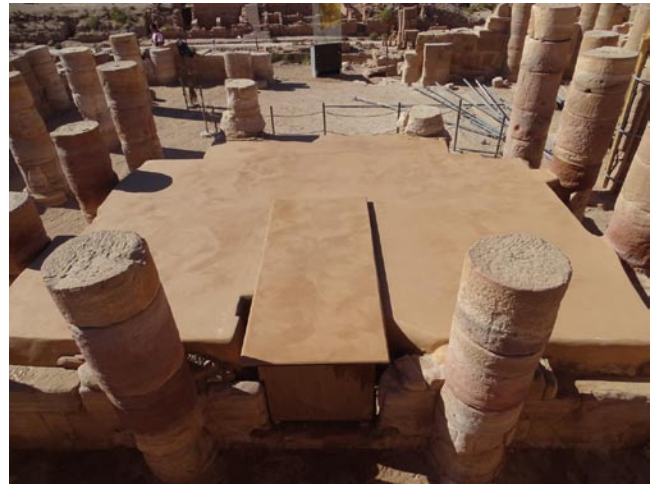
Before and after the application of a protective mortar capping on the cella podium (photos by Franco Sciorilli)
