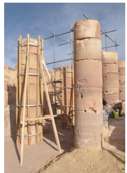
Columns in the west side of cella undergoing work led by Lead Conservator Franco Sciorilli with senior conservation assistant Hamza Wakhyan (left); TWLCRM documentation assistant Halemah Nawafleh applying mortar to a column (center); and one of the leaning columns after the addition of a wooden bracing structure (right) (all photos by TWLCRM team)
