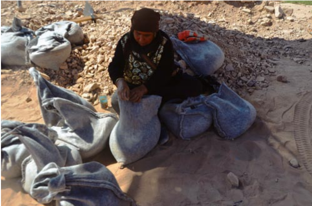
Team member Agelah Jmeidi stitching closed geotextile bags filled with sifted soil and rubble used to stabilize major on-site features (photo by Eman Abdessalam)
